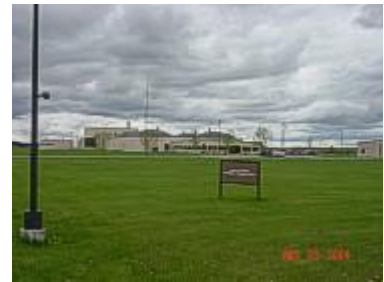
The Fargo and Moorhead wastewater treatment plants ensure that the levels of pathogens entering the Red River from discharges of treated wastewater are kept at a safe level.
